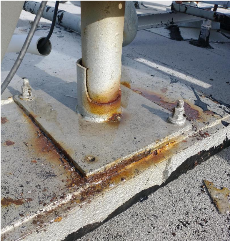
Tower mounting plate with two bolts and tower receiving cup
