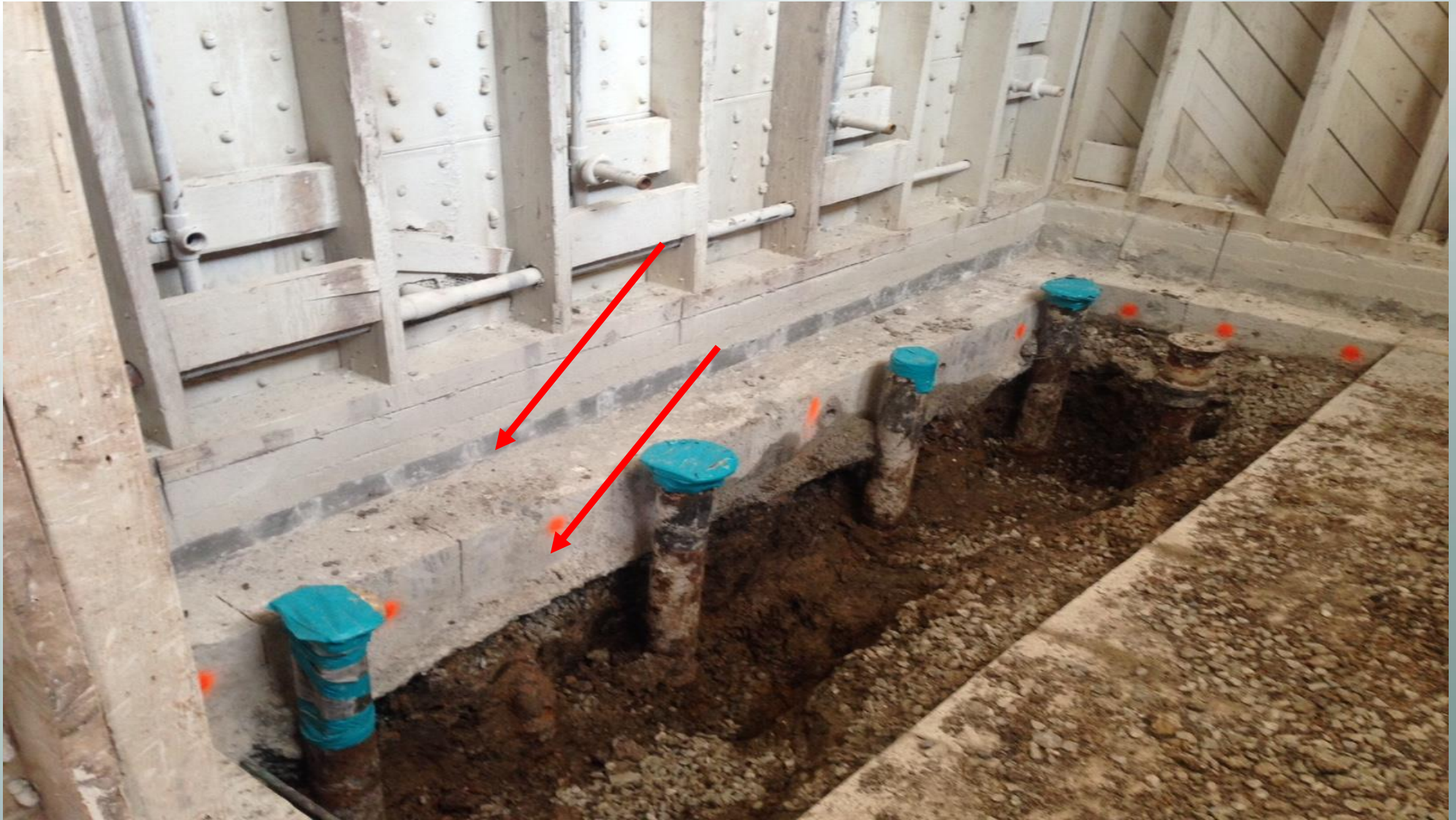
Concrete Slab – Riverview MS
