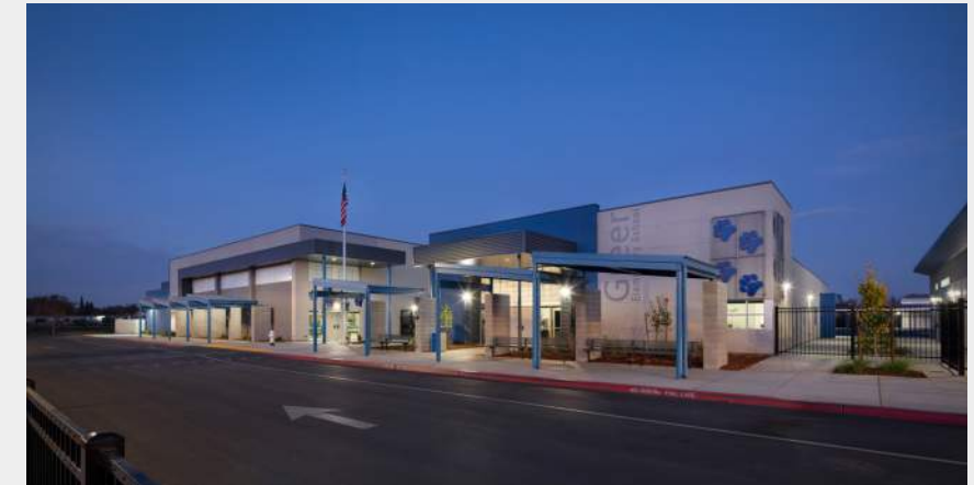
CHALLENGING PROJECT: SAN JUAN USD GREER ELEMENTARY SCHOOL
