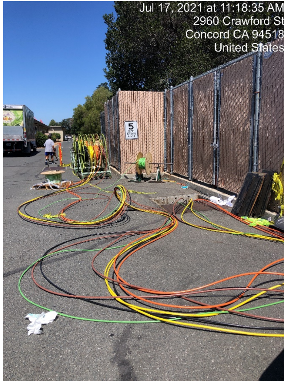
500 mcm laid out at main switch gear and Pt A
