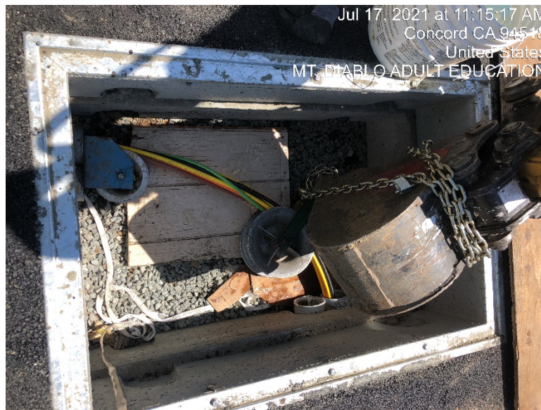
Set up for pulling cable with 45 degree radius bend
