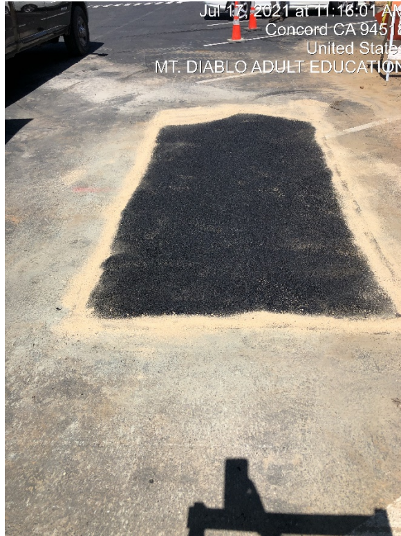
Asphalt patch back where conduit was repaired (2 locations)
