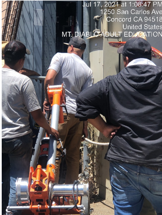
Setting up tugging and pulleys
