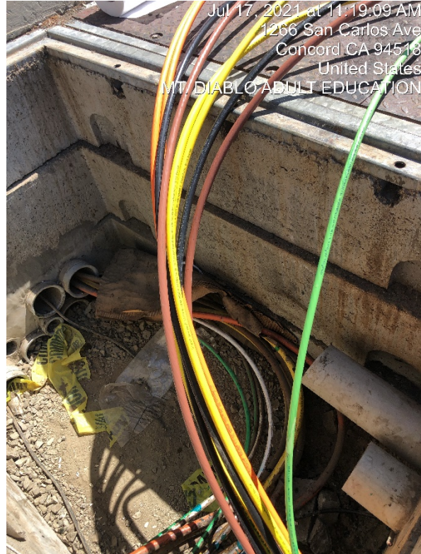
Cable for the new circuits (2)
