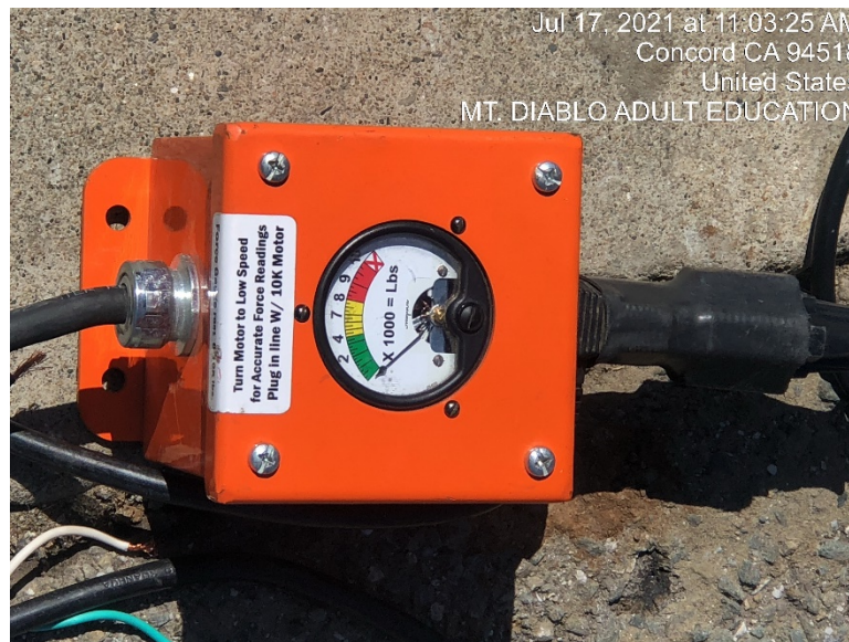
Force meter to monitor force during pulling
